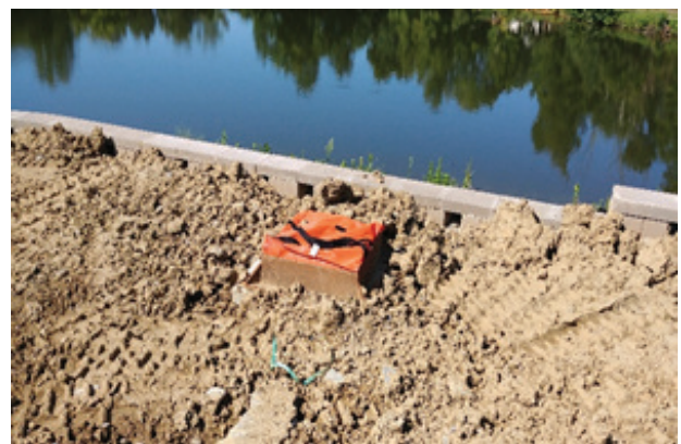
Catch basin inlet cover installed
