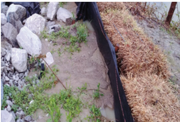
Rock berm, silt fence and straw bale system
