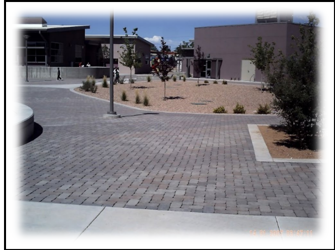
Permeable pavement and bioretention in Albuquerque, New Mexico (Photo courtesy of AridLID.org)
