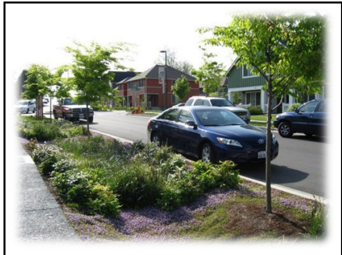
Street-side swale and pervious concrete sidewalk in Seattle, Washington (Credit: Abby Hall/EPA)
